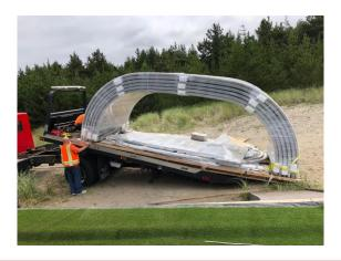
Warning – Tow truck bed should be at least as long as pallet to prevent damage. Pallet dimensions will be provided prior to delivery
